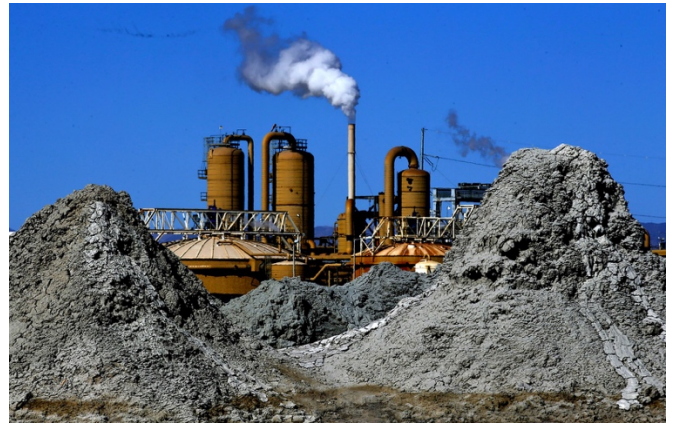
A GEOTHERMAL PLANT near the Salton Sea. The state now gets one-third of its electricity from renewable sources, and state law requires 100% climate-friendly energy by 2045. (Mark Boster Los Angeles Times)
