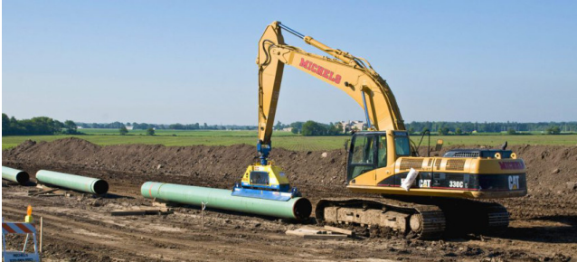
Pipeline construction. (photo: Education Images/Getty)
