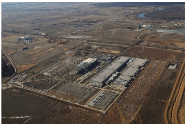
Google's energy-hungry data centers could become more expensive to cool its parent company has said. Above, a Google data center facility in Iowa. Credit Brian Snyder/Reuters
