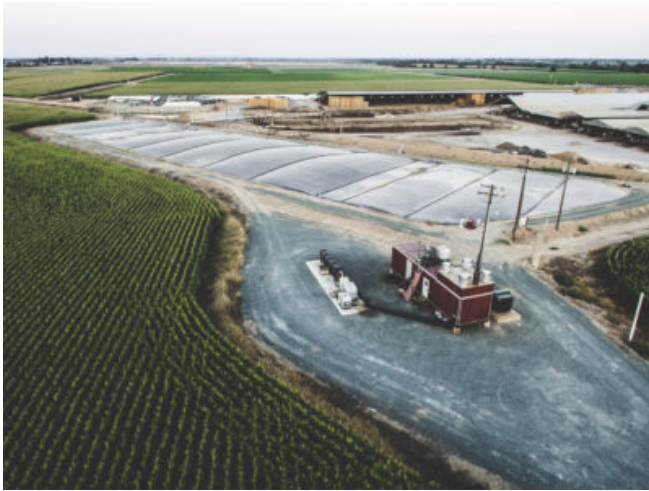
A covered lagoon manure digester on Van Warmerdam Dairy in Galt, California. Maas Energy Works
