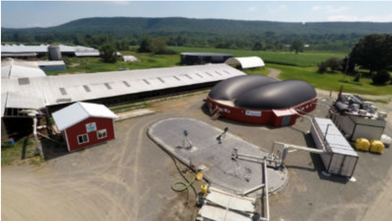
A manure and food waste-to-energy facility at Bar-Way Farm in Deerfield, Massachusetts. Vanguard Renewables
