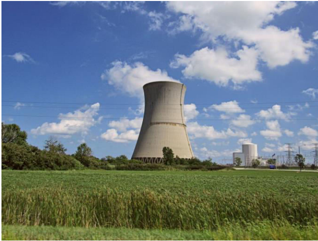
The Davis-Besse nuclear power station No. 1 in Ottawa County, Ohio Shutterstock
