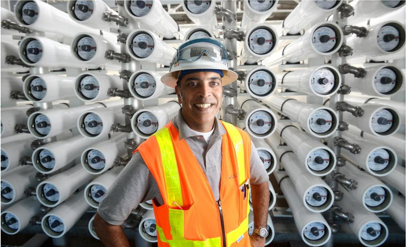
Mehul Patel is program manager for the Orange County Water District's Groundwater Replenishment System. He's standing amid vessels that use reverse osmosis membranes to filter treated wastewater and produce purified water. BILL ALKOFER, STAFF PHOTOGRAPHER
