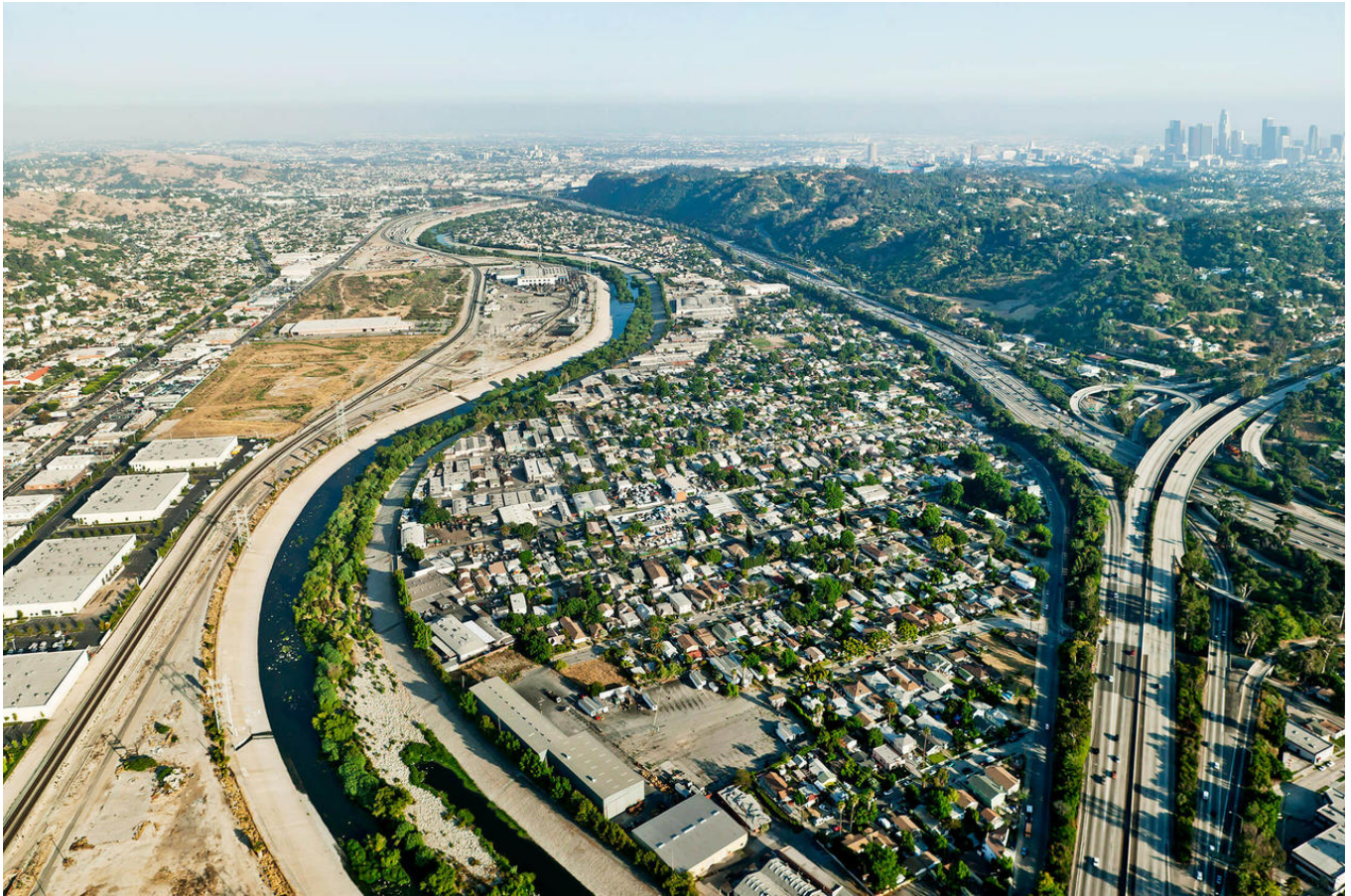
The Los Angeles River Lane Barden
