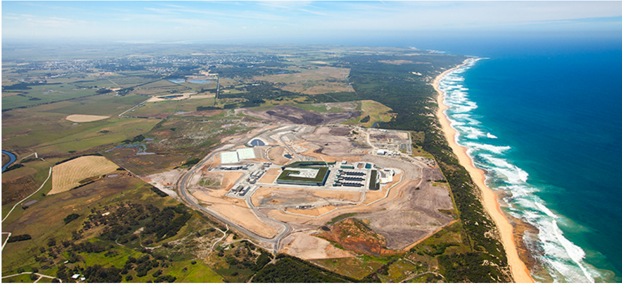
Desalination plant in Australia. (photo: unknown)
