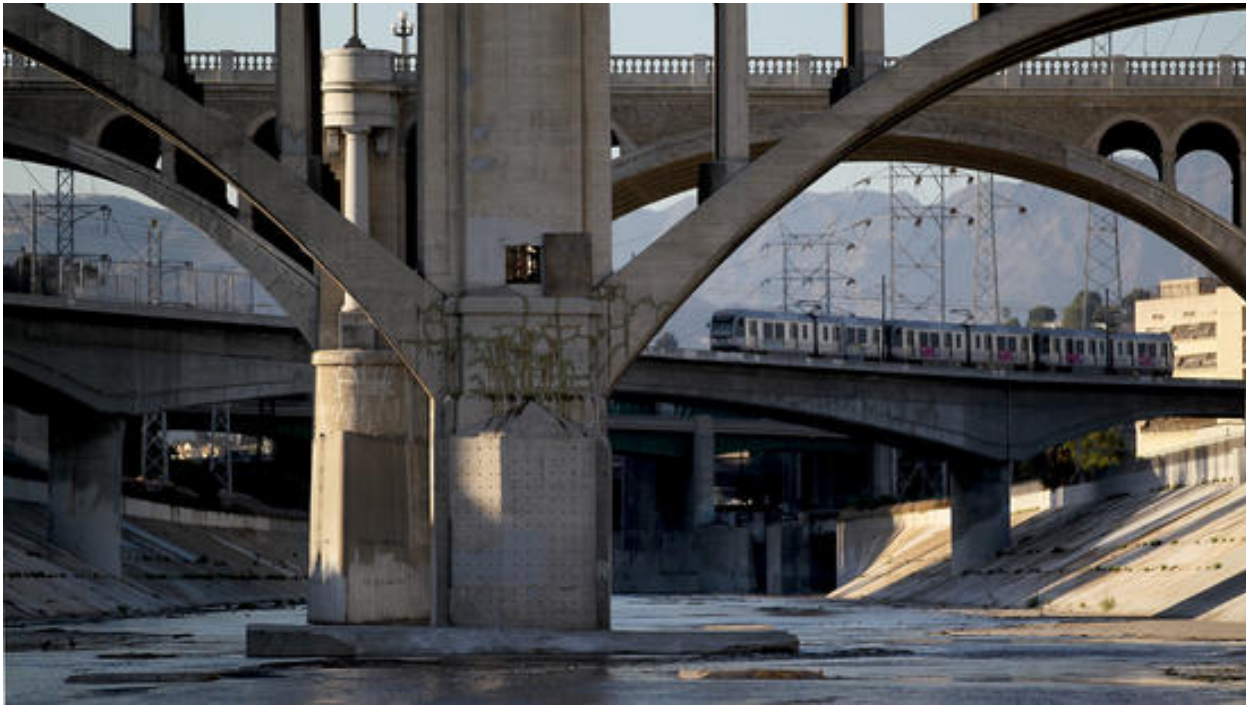
A Metro Gold Line train crosses the Los Angeles River near downtown L.A. (Luis Sinco / Los Angeles Times)
